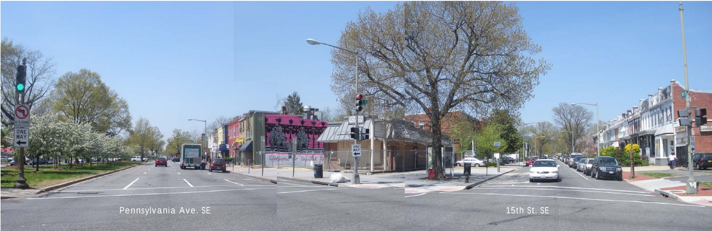
Site Panorama: view west @ intersection of Pennsylvania Avenue and 15th Street, SE
