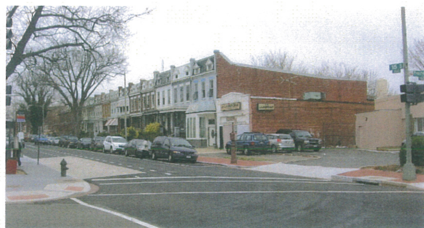
2 CORNER OF 15TH AND PENNSYLVANIA LOOKING NORTHEAST
